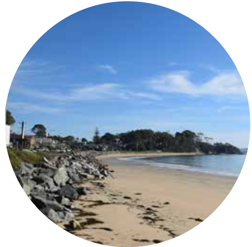
Rock wall (Caseys Beach)
