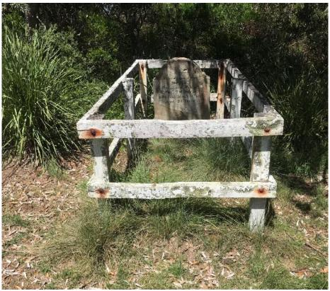
Photo showing active rust in the bolts and some timber splitting around the bolts. PG December 2017
