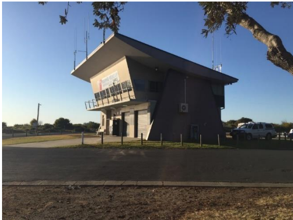
Marine Rescue building
