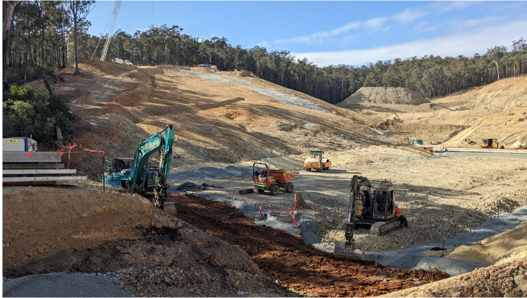
Dam wall under construction at the time of the site inspection
