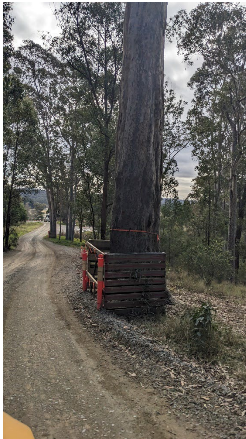
Vegetation protection measures in place on the compound access road
