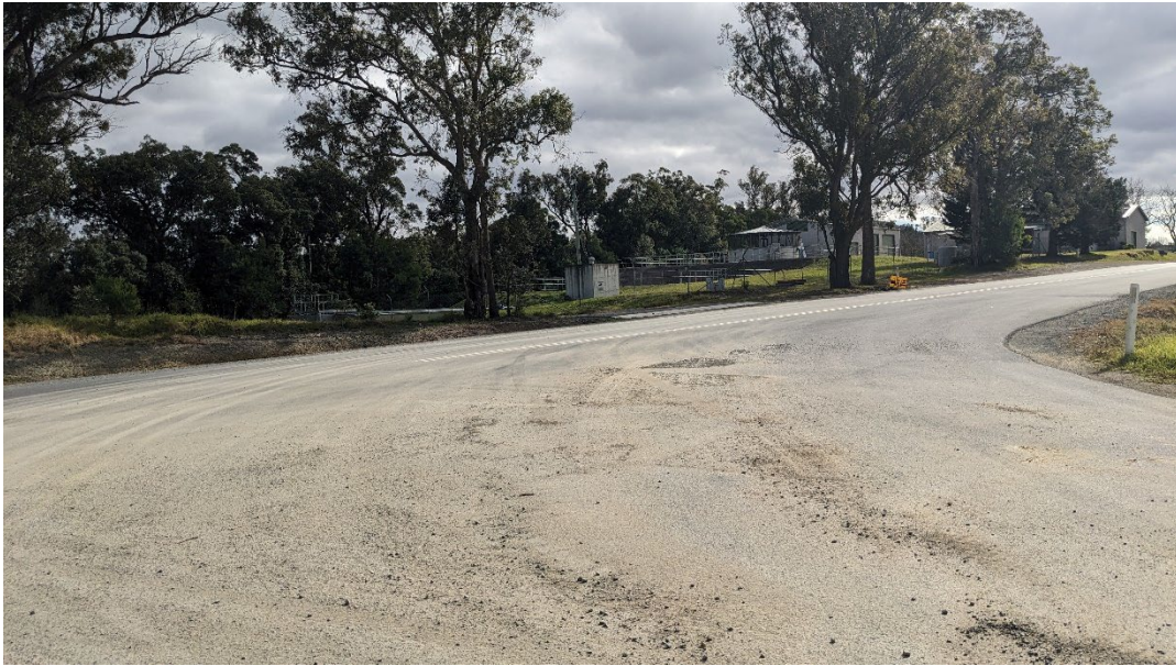
Minor amount of tracked material at the site intersection with Eurobodalla Road
