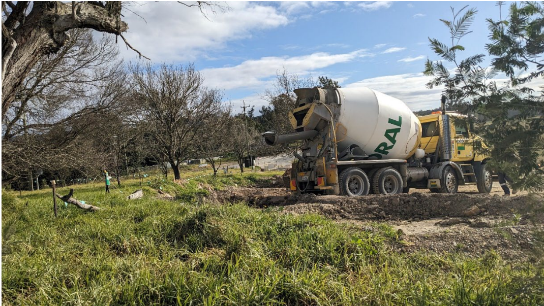
Dedicated concrete washout in place and in use
