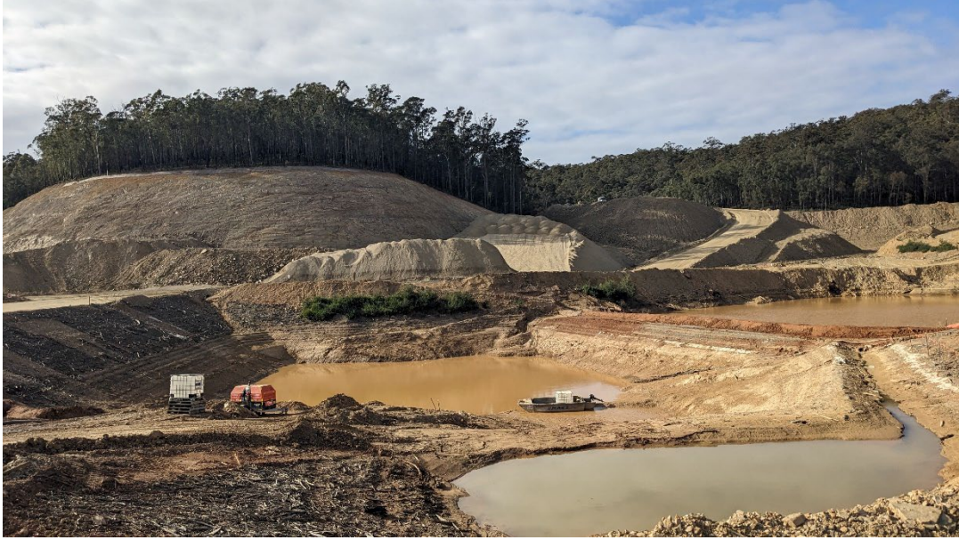
Coffer dam in place at the time of the site inspection
