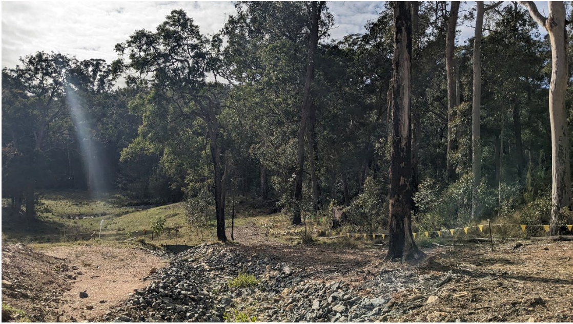
Heritage exclusion flagging and sediment controls in place
