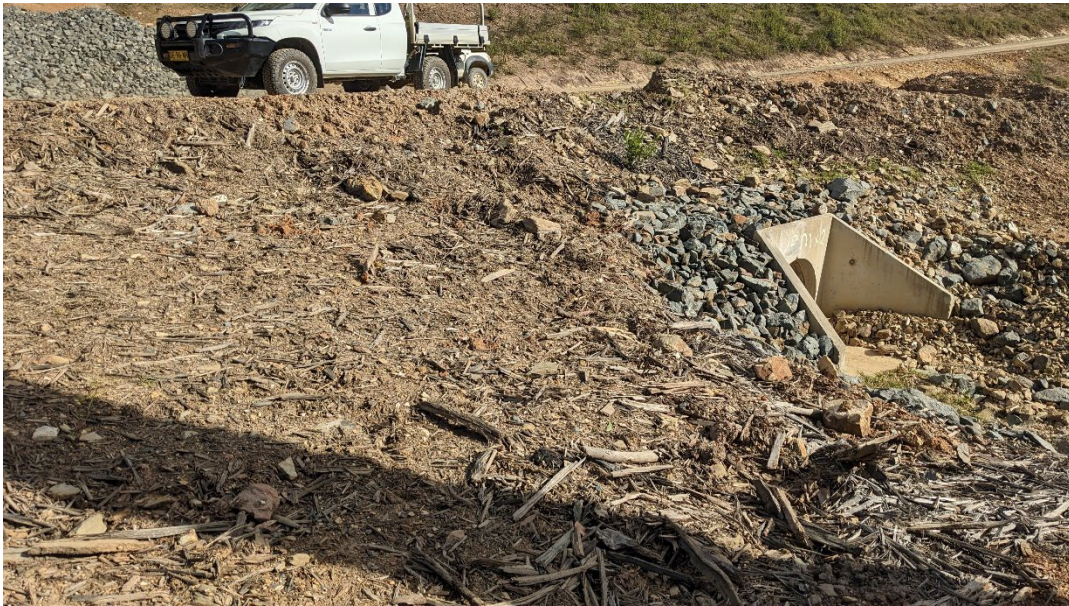
Mulch blanket applied to disturbed batters
