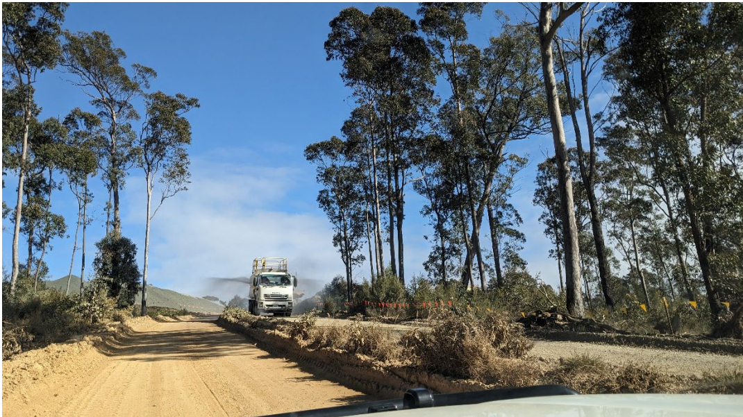
Water cart undertaking dust suppression on internal access roads
