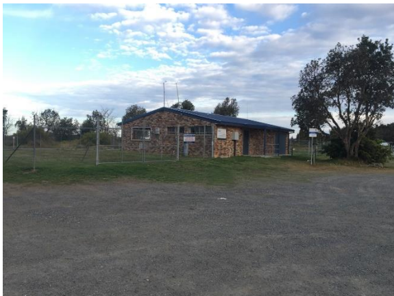
Sailing Club building, Hanging Rock Sporting Complex
