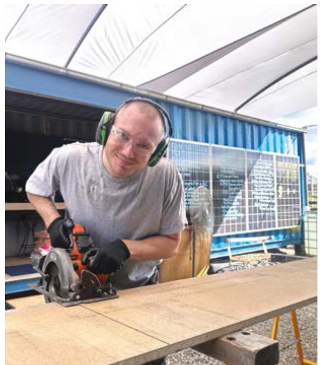
Image: Electrical apprentice Beau Cleary working in the Repurposing for Resilience space at the Moruya Transfer Station.
