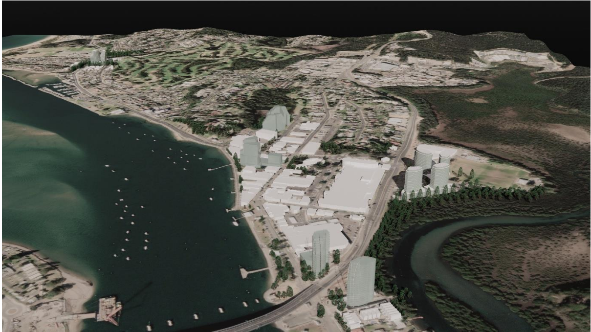
Figure 6– Aerial view from the northeast of the study area
