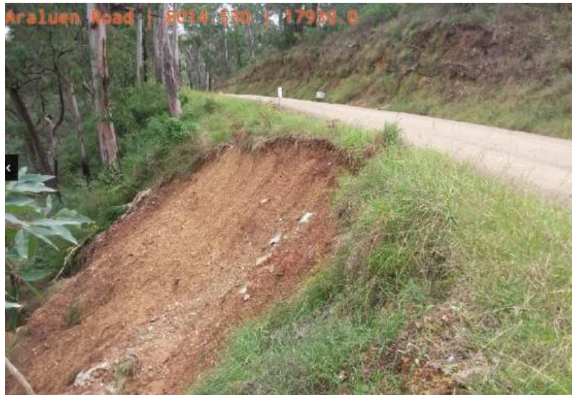
Figure 25: Existing Site Conditions DM02267
