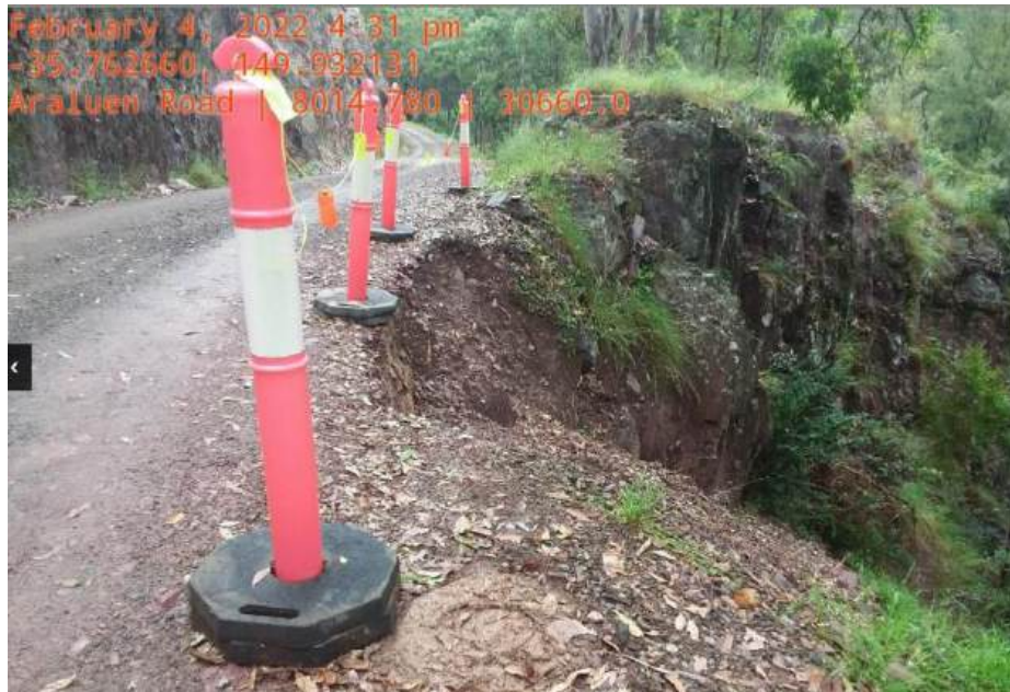
Figure 15: Existing Site Conditions DM01314
