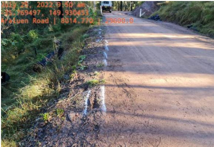
Figure 27: Existing Site Conditions DW00340
