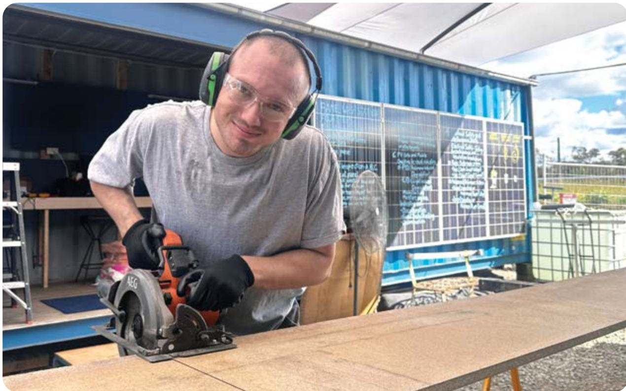
SAW SOLAR: Electrical apprentice Beau Cleary working in the Repurposing for Resilience space at the Moruya Transfer Station.
