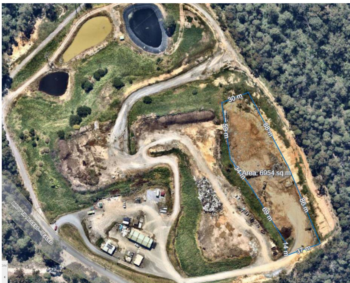
Figure 1-3: Existing Landfill Cell Area
