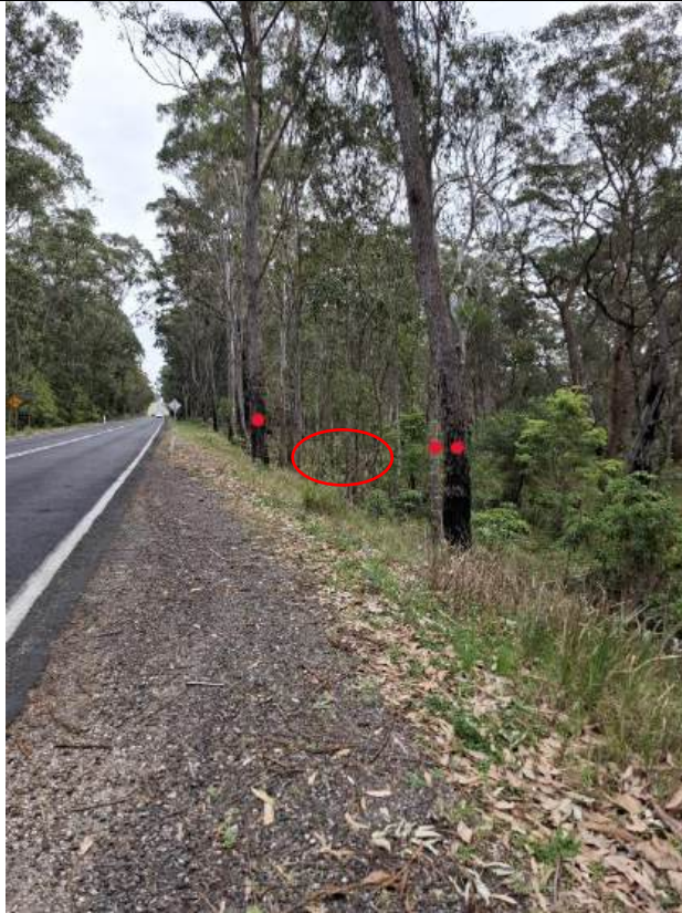
Figure 7. Photo showing the 3 young regrowth trees (marked by a red dot) and 5 saplings (circled in red) within the road batter to be removed. Trees to be marked clearly with an X prior to removal, and removed following all conditions in this REF.
