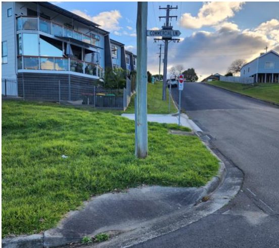
Figure 16: No footpaths and steep rise on Camp Street
