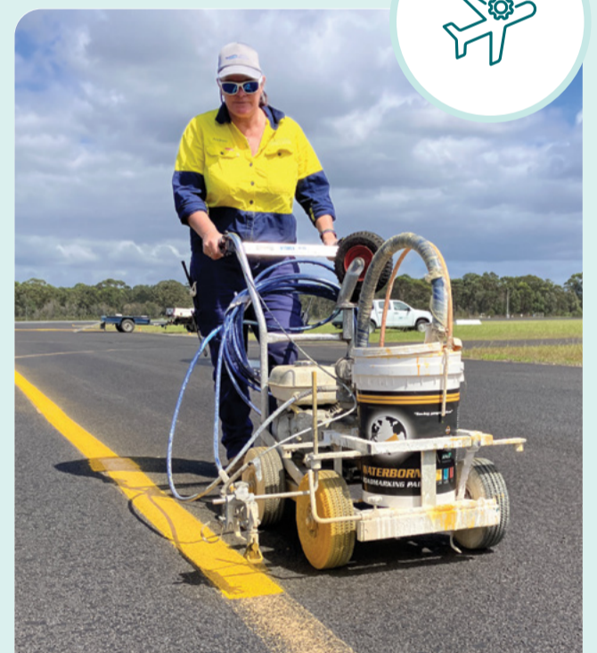
YELLA: Our airport coordinator Andy Dobson took charge of repainting many of the guidance lines at Moruya Airport.
